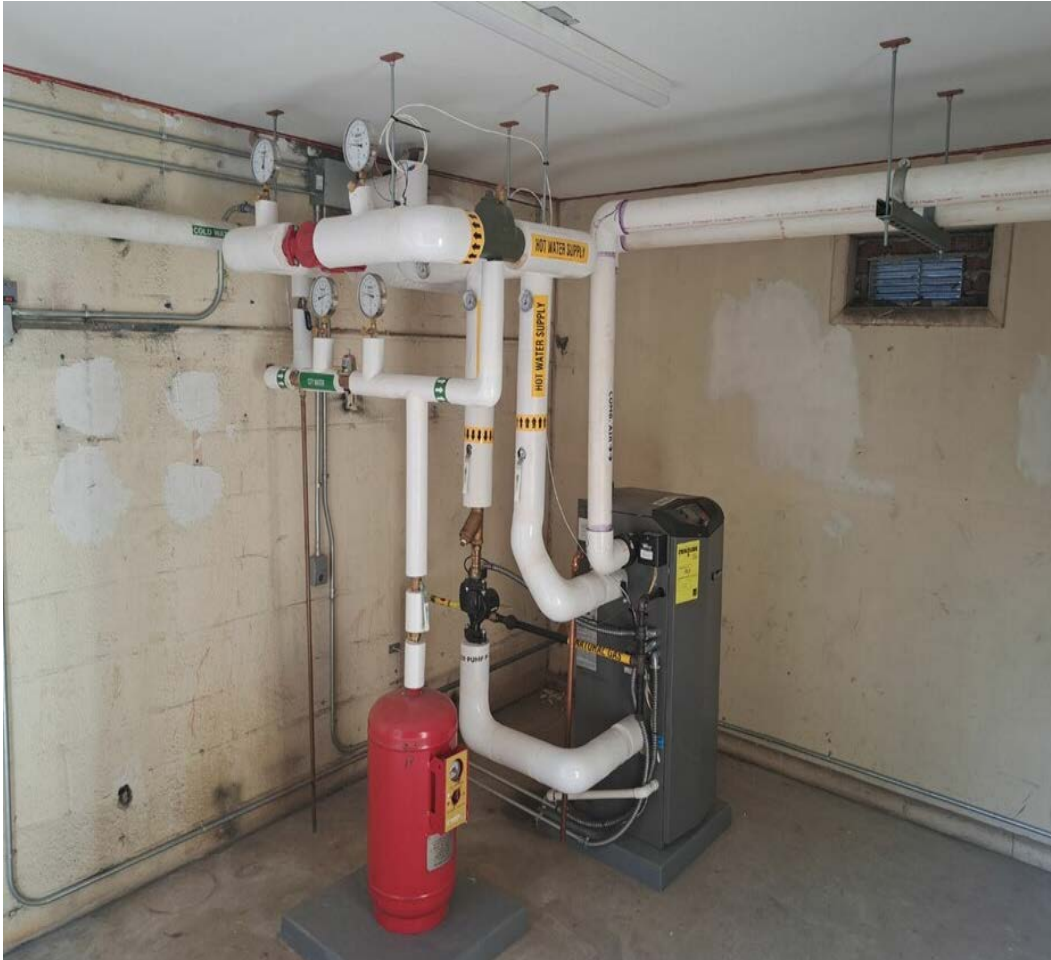
New Boilers Installed
