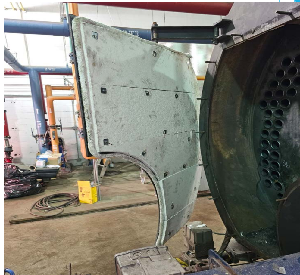
Completed Retubing/Refurbish
